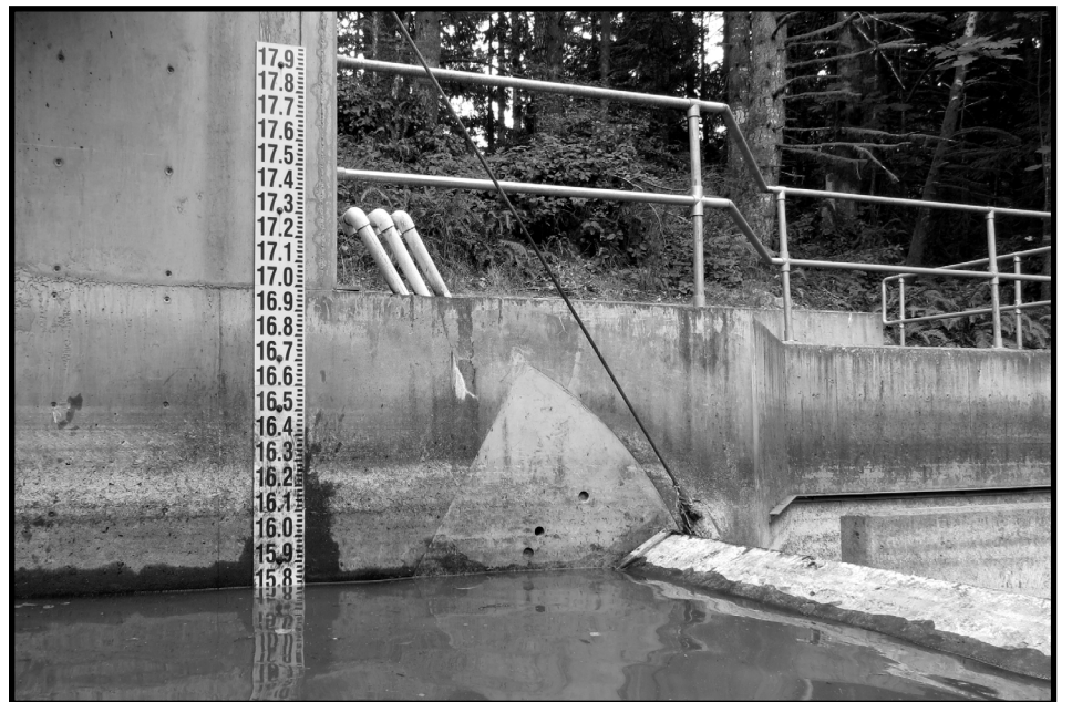
Current water level on the gauge at the weir is 15.81, or 115.81 metres above sea level.
