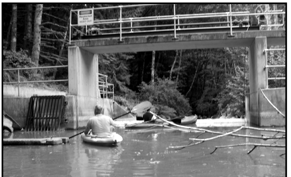
New weir. Fish ladder on the left, controls on top.
