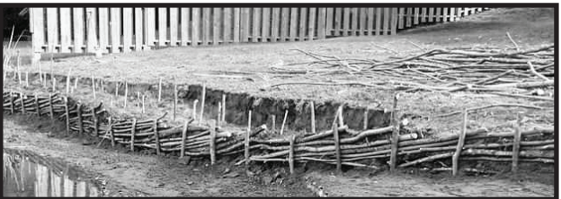
2-Start: Initial wattle wall with bulrushes.
