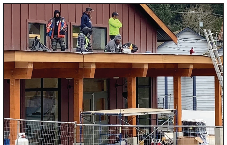
Putting the finishing touches on the Timber Canopy Roof
