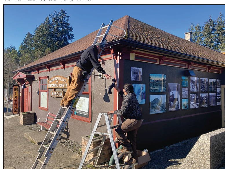
Gutters R US techs finishing up the gutter installation
