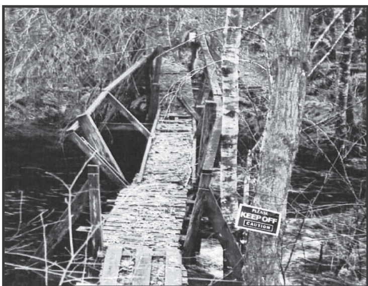
Old 1964 Dam & Walkway
